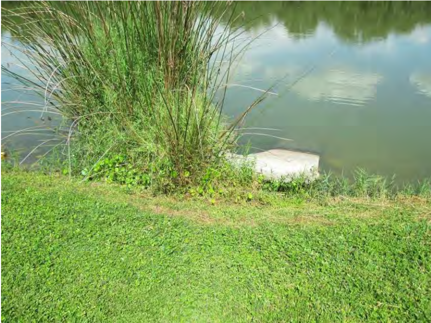
Lake 11- undermined MES & excessive vegetation on southwest bank
